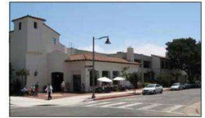
Above: View of Lined Building type from sidewalk showing a forecourt entry to the garage with the exterior building masking the interior building. Exterior building may consist of separate volumes as shown above in compliance with zone standards.
