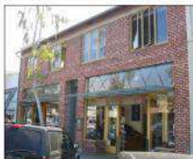
Example Main Street Commercial style building with classic floor-to-ceiling columns, shown on the ground floor using stone or masonry.
