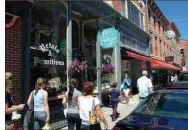
Shopfront Example - large glazing area of display windows, the bulkhead under windows, glass door, clerestory and shade awning.
